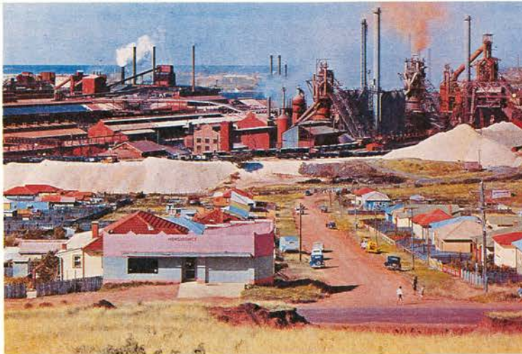
Forlorn suburban development in the shadow of the Port Kembla steelworks, c1955. Australia's preoccupation with industrial growth in the 1950s is evident in this placemat.
